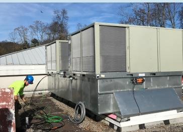
When an MSC client decided it was time to replace their thirty-yearold 40-ton rooftop unit, they wanted to build in some redundancy with the replacement. Because an in-kind RTU replacement does not exist, and a custom-manufactured unit would far exceed the customer's budget, our solution was to replace the 40-ton RTU with two 20-ton units ducted into separate areas and installed on a custom curb adapter designed to accommodate both units.
