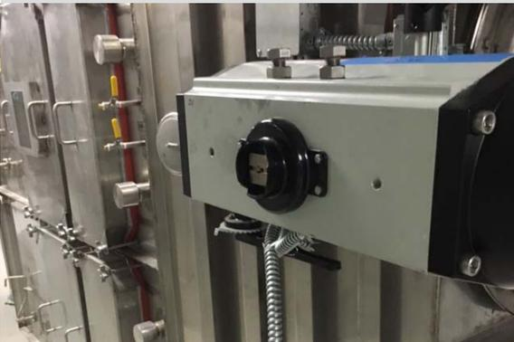
MSC responded to a service call for an HVAC system that wouldn't restart. Cooling was down and immediate help was needed. MSC quickly traced the problem to one of two dozen dampers. The damper had reopened properly but the limit switch was not closing the circuit. With minor mechanical linkage adjustments, the technician was able to adjust the linkage to get the limit switch to close when the damper was fully open. The control damper was retested and cooling restored.
