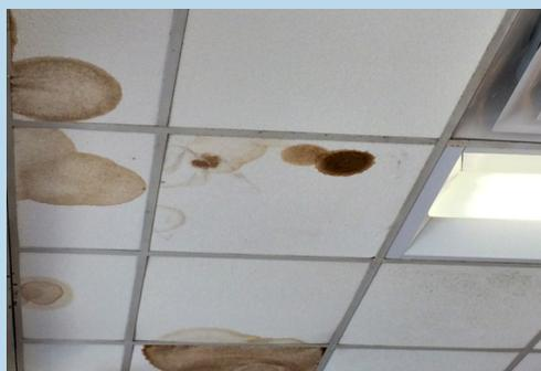
A new PM customer asked MSC to look into ceiling tile water stains in the conference room. Building staff had been unable to tell whether there was a roof leak or an exhaust duct was sweating. Our technician found the uninsulated duct to be dry to the touch, but using a psychrometric chart, he was able to determine that the duct would reach dewpoint on hot, humid days, causing condensation to drip onto the ceiling. Duct insulation and new tiles solved the problem.
