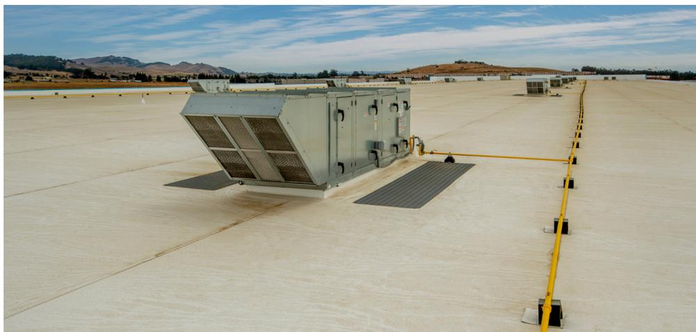
**T**he airside economizer is a mechanical device that draws in fresh outside air when temperatures are cool enough, enabling building owners to take advantage of free cooling and improve indoor air quality. Economizers are extremely effective in reducing energy costs, often to the tune of hundreds or even thousands of dollars a month, and are required by code in most commercial buildings.
