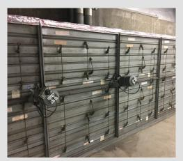
On a recent service call, our tech found low- and no-air conditions causing increased temps and occupant discomfort. Airflow static pressure and DP checks revealed issues in multiple dampers throughout the facility including bound linkage and blades, broken shafts, and non-operating actuators. Some dampers and actuators required replacement while others only required minor repairs. Damper testing and air balancing restored building systems to design intent.
