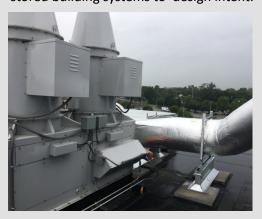
A hospital called MSC to investigate intermittent vibration and noise in a large exhaust fan. After running the fan through various speeds, it became evident that the rotating fan shaft was creating **resonant vibrations** as it passed through critical speed at 41 to 43 Hz. We programmed the drive to pass quickly through this band to prevent damage while accurately maintaining negative static pressure.
