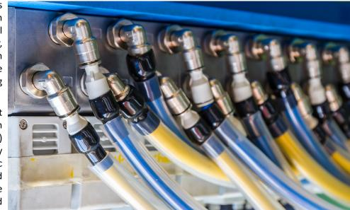
proper operation of pneumatic controls depends on dry air in the tubing as well as transducer and positioner accuracy. Bladders, springs, and diaphragms all require annual calibration, inspection, testing and leak checking as they have a tendency to drift out.
