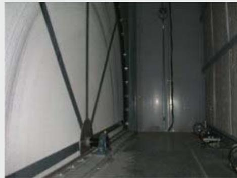
When MSC was called in by a client to address temperature complaints, technicians quickly zeroed in on several 11 year-old heat recovery wheels. This led to analyses of operating conditions, bearings, seals, casing drives and sensors to identify specific problems. One of the issues uncovered was the bypass of air through seals between supply and exhaust. *Continued On Page 2*
