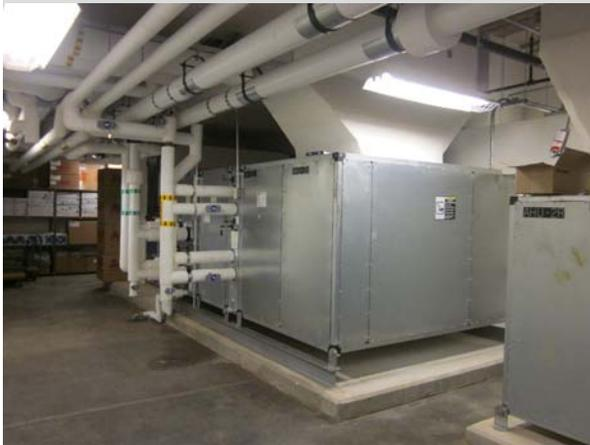
**MSC installed data loggers** to test temperature sensor accuracy in response to a high temp complaint. The sensors were found to be off by 2°-4° and required calibration. Sensors require annual calibration, but maintenance personnel had allowed 19 months to elapse. MSC also replaced a failed RH sensor with a factory-calibrated device, as well as several neglected HEPA filters and pre-filters, illustrating the importance of proper PM.
