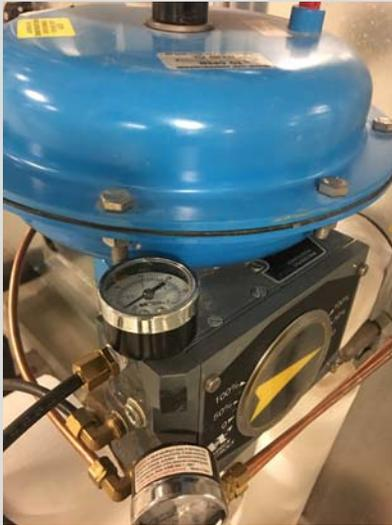
**Lightning Power Failure** - An emergency call came in to MSC when a hospital lost power during a thunderstorm. Emergency power came online within seconds, but backup emergency exhaust failed to start due to loose damper linkage and slightly-undersized actuators. MSC replaced the old, sloppy mechanical linkage with Belimo direct drive actuators.
