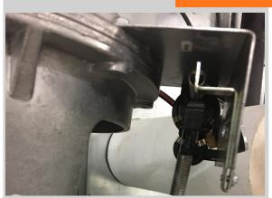
Bad Valve Modifications – MSC was called to a project to troubleshoot multiple malfunctioning humidifier control valves, making it impossible to properly control RH in lab spaces. Upon inspection, we discovered that someone (who clearly didn't know what they were doing) had cut, bent, and reinstalled the original control valve positioner springs on all eight valves. New springs were shipped overnight, installed and properly calibrated, returning the labs to proper humidity control.
