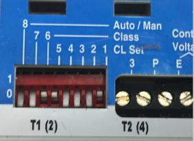
Dip-Switch Settings — A new motor control center was installed for a longtime customer and MSC came in to assist the electrical contractor with commissioning. Condenser water pump starters were tripping and locking out, but everything appeared to be wired correctly. A check of the O&M manuals revealed that several of the dip switches controlling time delay were in the wrong position. The switches were reset, and the problem was quickly resolved.
