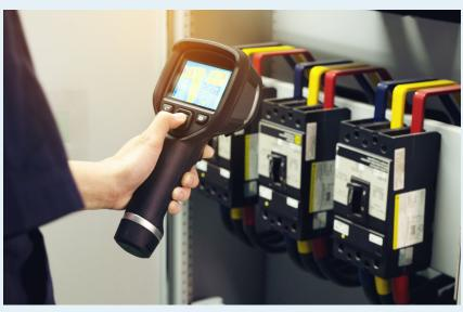
When electrical anomalies occur, loose, over-tightened, or corroded connections are often at the root of the problem. Effects of a bad connection can range from annoying (intermittent interruption) to costly (critical system failure), to catastrophic fire or explosion.
