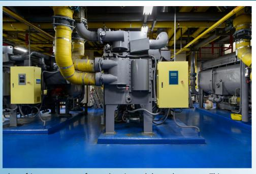
Pressure builds up in the compressor, causing the refrigerant to surge forward again, and the cycle repeats. This reverse-load can damage the thrust assembly, bearings and gearbox, and can cause a rupture in the safety disc or blow the relief valve.
