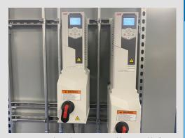
MSC received a no-cooling call from a lab where a bad connection on a chilled water pump VFD caused wiring and part of the drive to burn up. Despite ongoing pandemic supply issues, we located a 25 hp replacement drive and had it onsite within hours. We switched the system over to the lag pump, installed the new drive, and restored full cooling capabilities to the facility that same day. Both VFDS were tested and commissioned to ensure proper operation.
