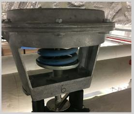
A fairly new facility called MSC with complaints about a chilled water control valve and possible coil flow issues. A visual check of chilled water valve movement showed that excess insulation was interfering with operation of the control valve positioner. Our technician also found that multiple discharge air temperature sensors had been recalibrated incorrectly and were off by 2F-8F. Insulation repairs and installation of new sensors corrected the problems.
