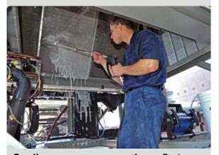
Cooling season preparation – Spring cleaning of chiller tubes, coils and cooling towers is vitally important to ensure proper system performance. Chilled water piping should be flushed annually with trisodium phosphate (TSP), then rinsed and filled with clean water. Strainer baskets should be thoroughly cleaned as well. Use a corrosion inhibitor to protect pipe integrity, and be sure to vent air before operating the system.
