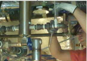
Steam Condensate Flooding- Managing steam condensate is very important, particularly when it comes to trim humidifiers. When designing and installing condensate piping, it is important to determine whether there will be any pressure to lift the condensate or if it needs to drain by gravity. Condensate flooding and water damage is a common occurrence when proper pipe requirements are not met.
