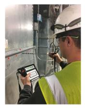
process suites. All VAV boxes on both supply and exhaust were tested, airflow-checked, and fine-tuned to maintain proper DP. We also discovered numerous automatic doors that were staying open too long or not fully closing against the air pressure, causing rooms to go into full-exhaust mode and triggering alarms.
