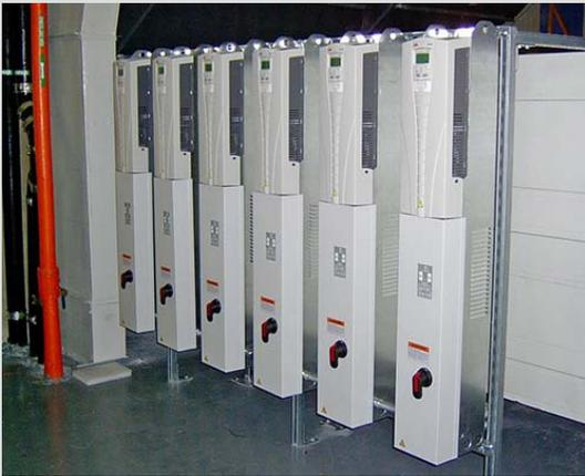
**VFD and Backup Cooling** - Cooling problem in walk-in boxes: condensers were served by a cooling tower, and drives for the tower water had shut down due to a voltage dip and failed to restart automatically. City water backup to the condensers also failed when the backup valve didn't open in time due to a programming error. Techs reprogrammed the drives to auto-start and corrected the backup system delay.
