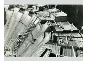
All concrete generates heat, and in mass placement the concrete can get extremely hot, affecting strength and durability. If the Hoover Dam was built in a continuous pour with no method of heat dissipation, it would have taken 125 years to cool to ambient temperatures, threatening structural integrity.
