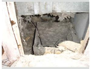
This dirty ductwork was found during a walkthrough at a new customer's facility. The previous contractor was supposed to have inspected filters and ductwork for cleanliness. It is not uncommon for us to come across such conditions. Make sure your PM is done, and done properly.
