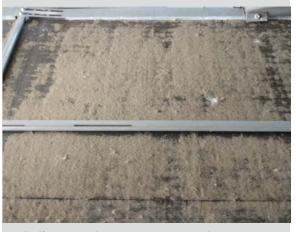
A dirty condenser cannot exchange heat properly. This will cause systems to run hot, significantly shortening the life of the equipment and raising energy costs. Simple follow-through maintenance can have a real impact on many fronts.
