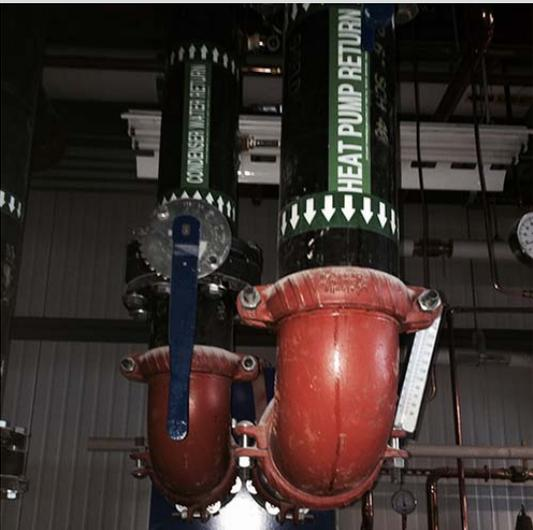
**Heat Pump** – Large heat pump loops depend on constant circulation for proper heat exchange. Problems with flow, heat exchangers, controls, or cooling towers can jeopardize the loop and shut off heat pumps. During a recent heat wave, a client's backup pump failed to come on during a power outage due to a controls issue, stopping circulation, tripping heat pumps, and shutting off cooling.
