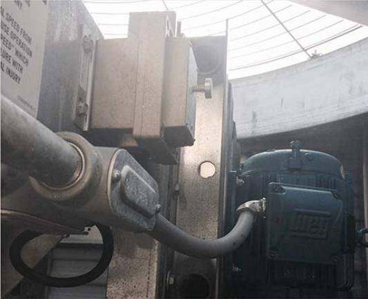
**Vibration Sensors** – Cooling tower vibration sensors monitor fans, gear housing, shafts and motors for excessive vibration and provide early warning before a catastrophic failure can occur. An MSC client's vibration sensor recently alerted them to a vibration issue that was traced to a bad bearing, and a costly tower failure was successfully averted.
