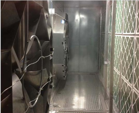
**Stratification** – Freezestat trips are oftentimes the result of poor or uneven heating coil sections, control valve issues, or stratification, which is the tendency of cold air and warm air to separate into layers. Freezestat trips can occur in air handling units when cold outside air and warm return air remain stratified and reach the freeze stat together. A blender should be designed and installed to properly mix the air to a uniform temperature.
