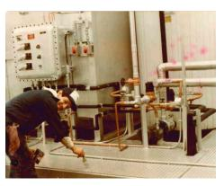
new explosion-proof bolts. The unit was a cascade refrigeration system utilizing R-502 refrigerant in the high stage and R-503 was used in the low stage to cool methylene chloride down to -100°F in order to condense the gasoline vapors. Both of these refrigerants were banned in 1995.
